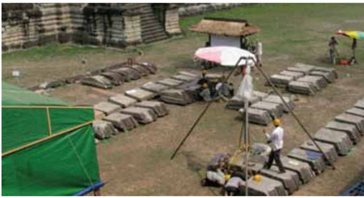
Figure 6: Stones removed from the Angkor Wat roof structure being conserved in the on-site workshop. Courtesy of the World Monuments Fund.
