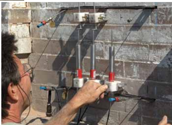
Figure 3: Measuring masonry compression response in place using the flatjack method of ASTM C 1197. Courtesy of Atkinson-Noland & Associates, Inc.
