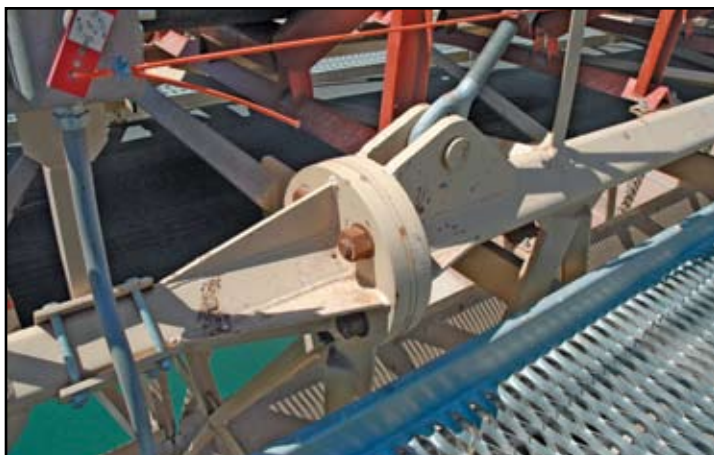
Figure 5: Typical vertical cable-to-truss connection.
