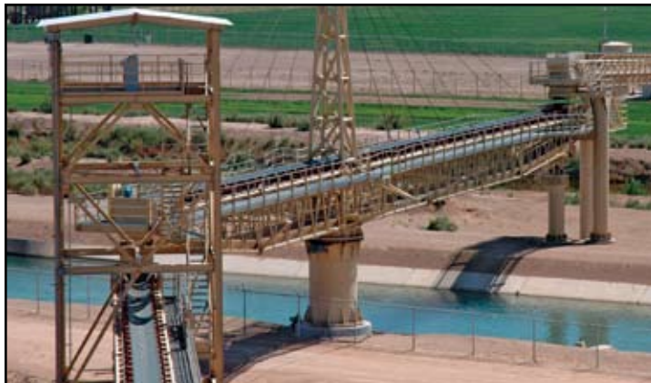
Figure 3: View of the conveyor belt system and control tower, looking south from the head end (U.S. side). The view shows the swing bridge conveyor belt system in the "Working" position.
