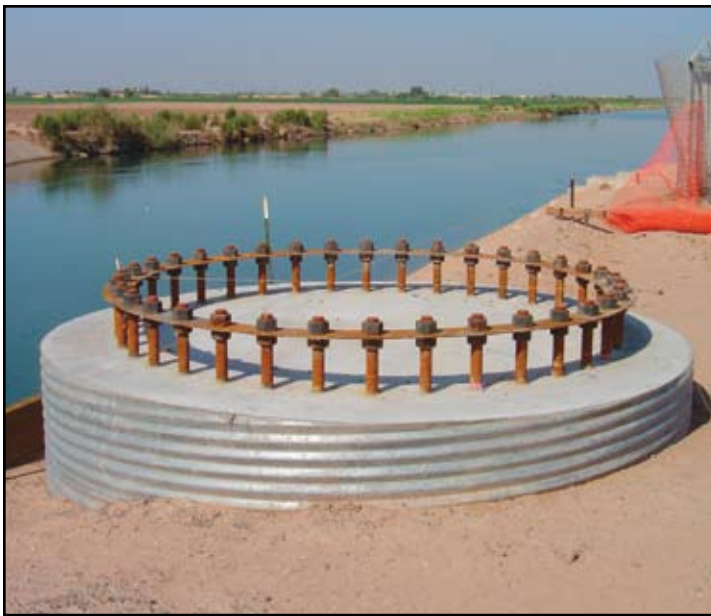
Figure 7: Drilled Shaft Support for Bridge Pivot.
