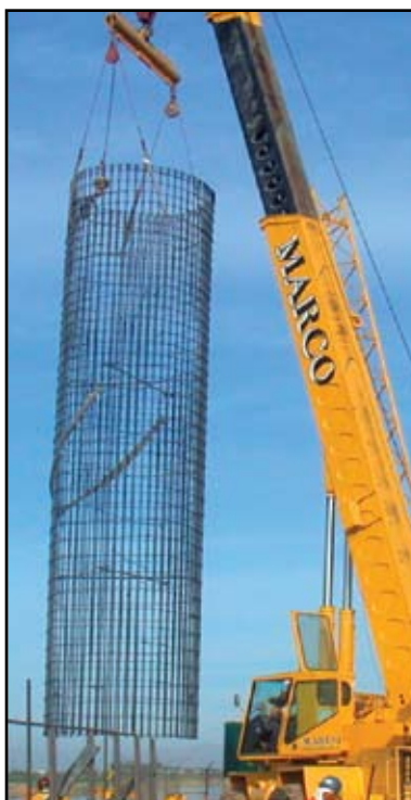
Figure 6: Installation of Drilled Shaft Reinforcing Cage for Bridge Pivot.
