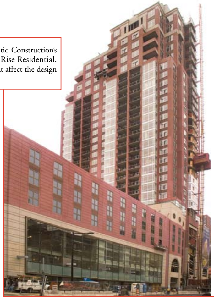
For the 24 residential floors of Symphony House, the developer chose light-weight architectural precast concrete panels.
