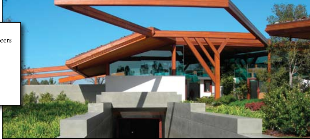
A tree column supports steel beams above the driveway. The driveway walls are finished in a unique concrete veneer with horizontal joints at 36 inches (no vertical joints). Courtesy of Norm Applebaum Architect, AIA.
