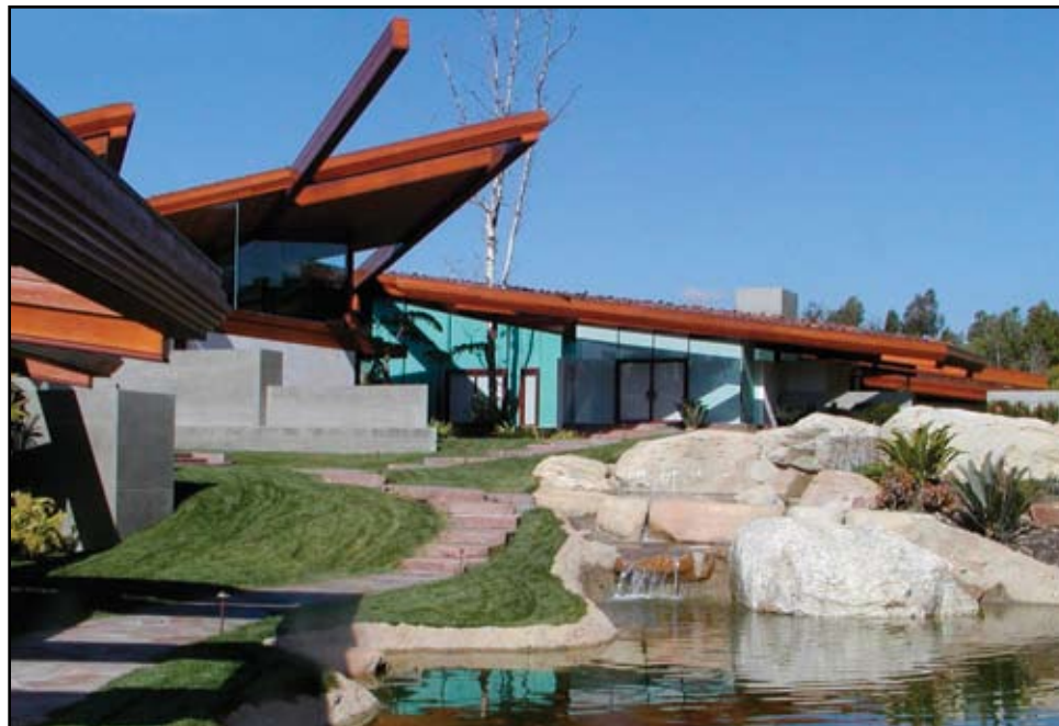
Steel beams infilled with Douglas fir create dramatic roof lines. Door frames are surrounded by glazing and constructed from solid steel plates cantilevered up from floor framing. Courtesy of Rose Nielsen.
