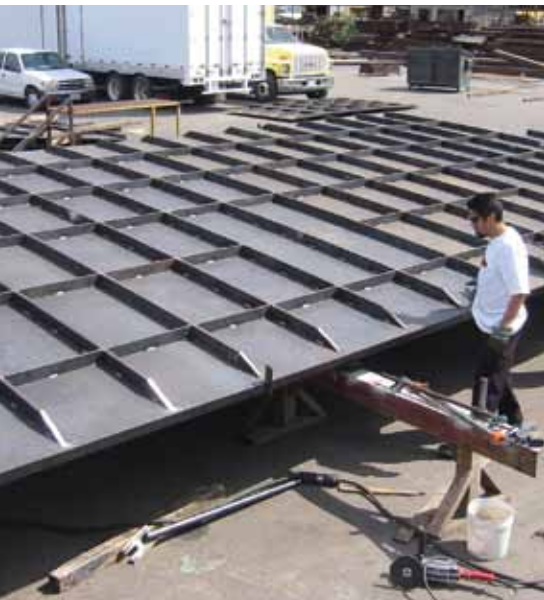
Segments of canopy during fabrication.
