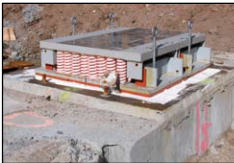
Figure 2: Spring isolator – subway tunnel.
