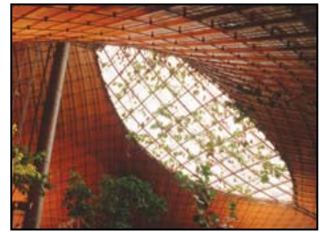
Cable-net clad with timber at the Institute for Lightweight Structures and Conceptual Design (ILEK), University of Stuttgart. Architect: Frei Otto. Courtesy of ILEK.
