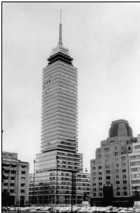
The Latino Americana Tower, Mexico City’s tallest high-rise. It has withstood several large magnitude earthquakes with little or no structural damage. Courtesy of Civil Engineering Department, University of Illinois.
