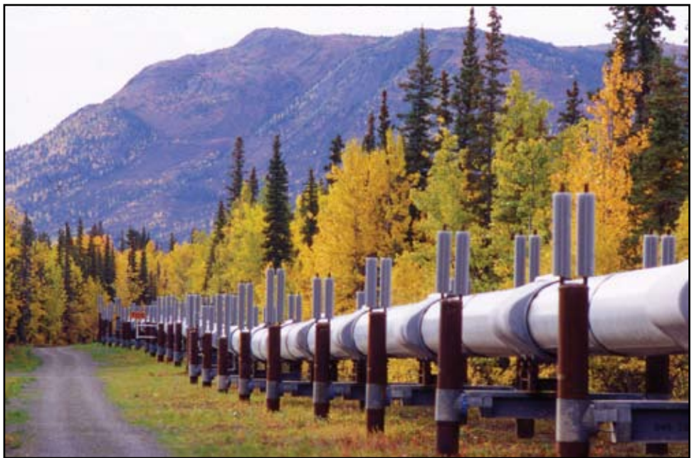
Elevation of Trans-Alaska Pipeline. Courtesy of Alyeska Pipeline Service Company.
