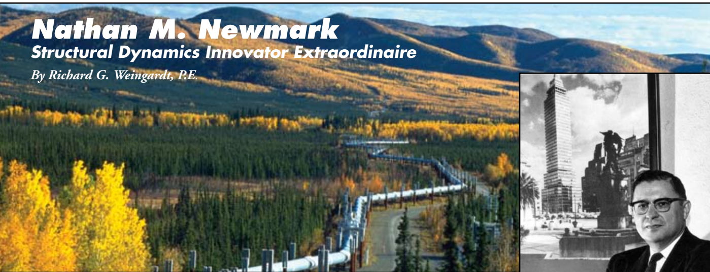
Trans-Alaska Pipeline in the fall. Courtesy of Alyeska Pipeline Service Company.
