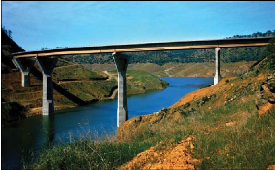
James E. Roberts Memorial Bridge.
