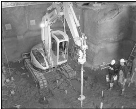
Figure 1: Helical Foundation Installation.
