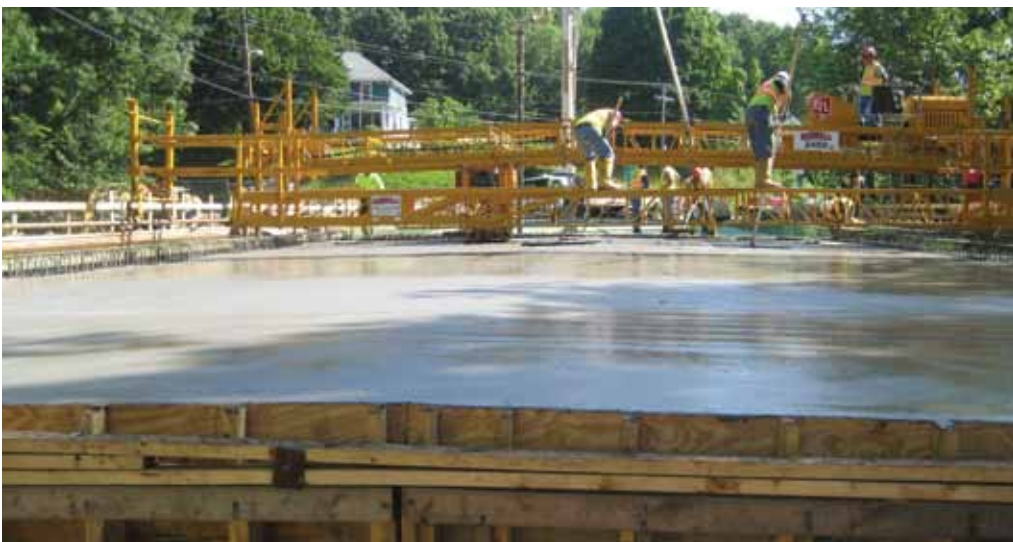
The bridge construction crew conducts the pour.
