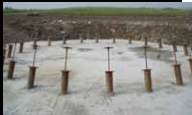
Figure 2: 24 micropiles installed and ready for the pile cap.
