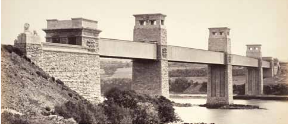
1850 Britannia wrought-iron tubular bridge over the Menai Strait. Courtesy of Los Angeles County Museum of Art.
