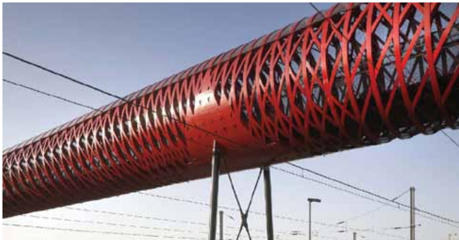
Tschumi-Dutton’s 2010 steel upgrade of Rogers’ 1841 timber design. Courtesy of Bernard Tschumi architects, Christian Richters, photographer.
