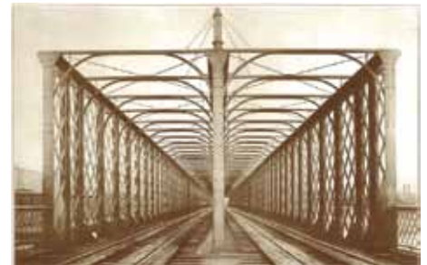
Figure 6: Pittsburgh, Fort Wayne & Chicago Railway. Rider's lattice configuration, wrought-iron truss. Built in 1868 over the Allegheny River near Pittsburgh, Pennsylvania. (Courtesy, Pittsburgh History and Landmarks Foundation.)
