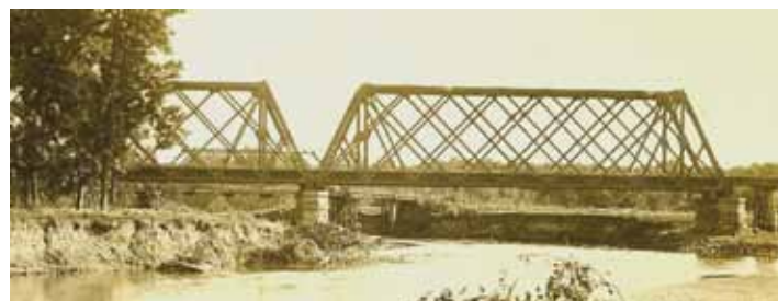
Figure 2: Typical Metal Lattice Railroad Bridge. Over the Coon River, Lake City, Iowa. (Author's post card collection.)
