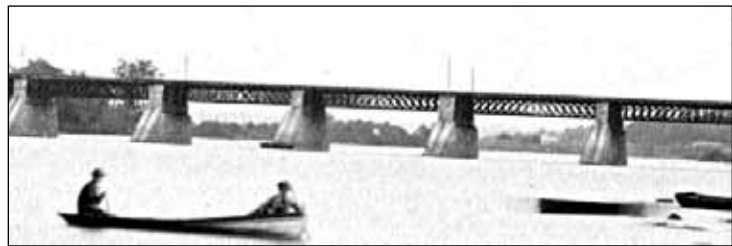
Figure 7: Carroll's 1859 Bridge over the Mohawk River between Schenectady and Scotia, New York. (Courtesy of Schenectady Historical Society. Provided by Katherine Chansky.)
