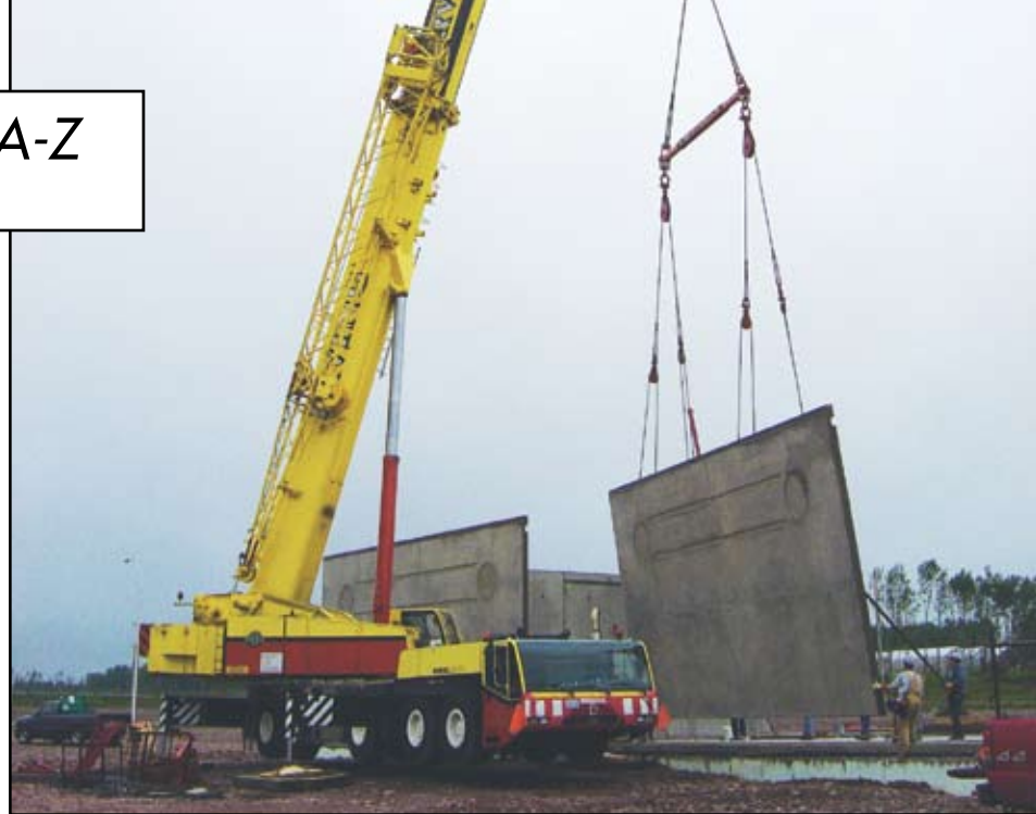
200-ton truck mounted hydraulic boom crane lifting 43,000-pound panel.
