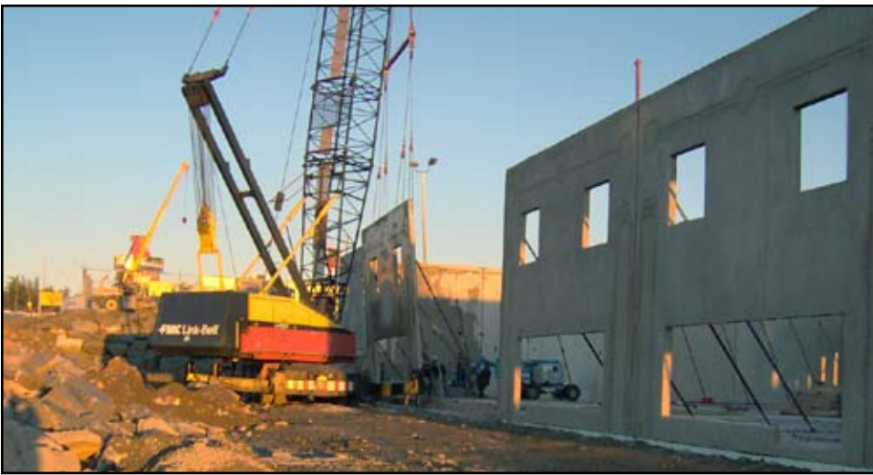
Conventional 200-ton truck mounted lattice boom crane lifting 52,000-pound panel.
