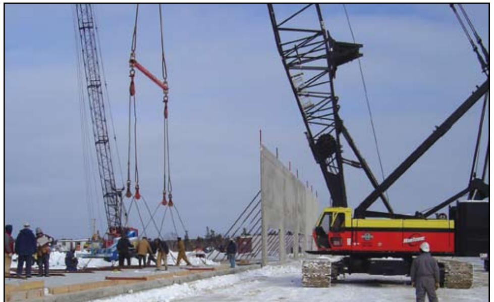
230-ton track mounted lattice boom crane lifting 80,400-pound panels.
