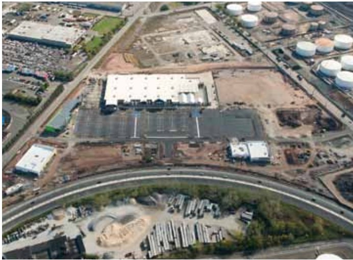
Aerial photograph of the completed Essington Produce Market Warehouse. Courtesy of R. Alan Adams Photography.
