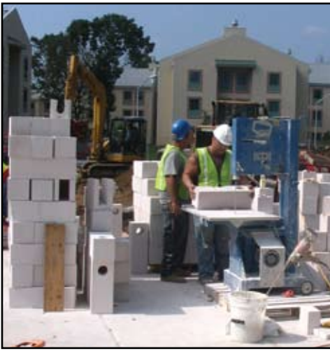
AAC is cut to size using a band saw.
